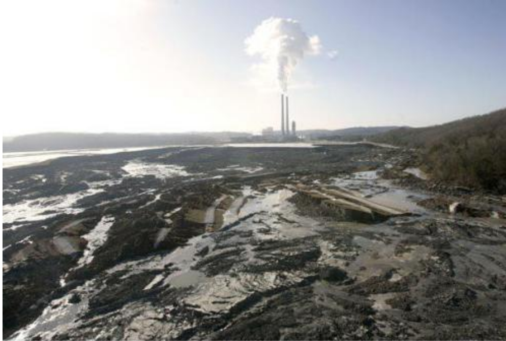
Aftermath of a retention-pond-wall collapse
