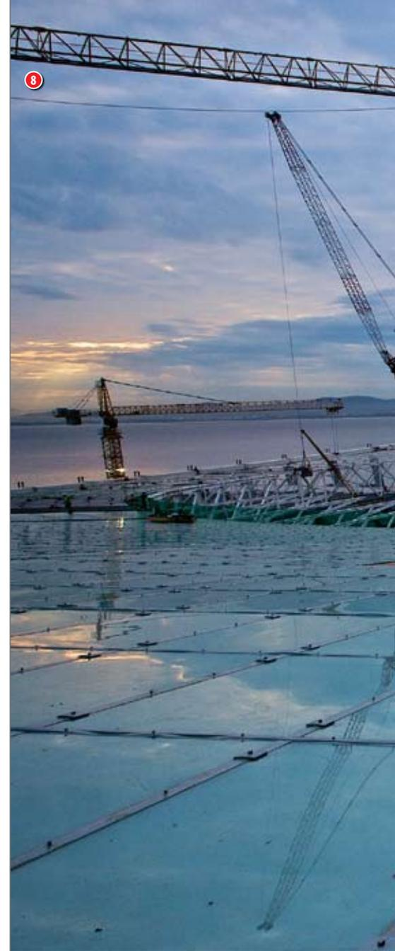
The higher-than-expected tender prices prompted a cost-cutting exercise, resulting in the reduction of the width of the bowl around the pitch, making the 72 radial frames less stiff. The inclined pylon columns supporting the roof were revised in cross-section from 6 m x 1 m to 3 m x 0,8 m, severely reducing bending capacity and stiffness.
