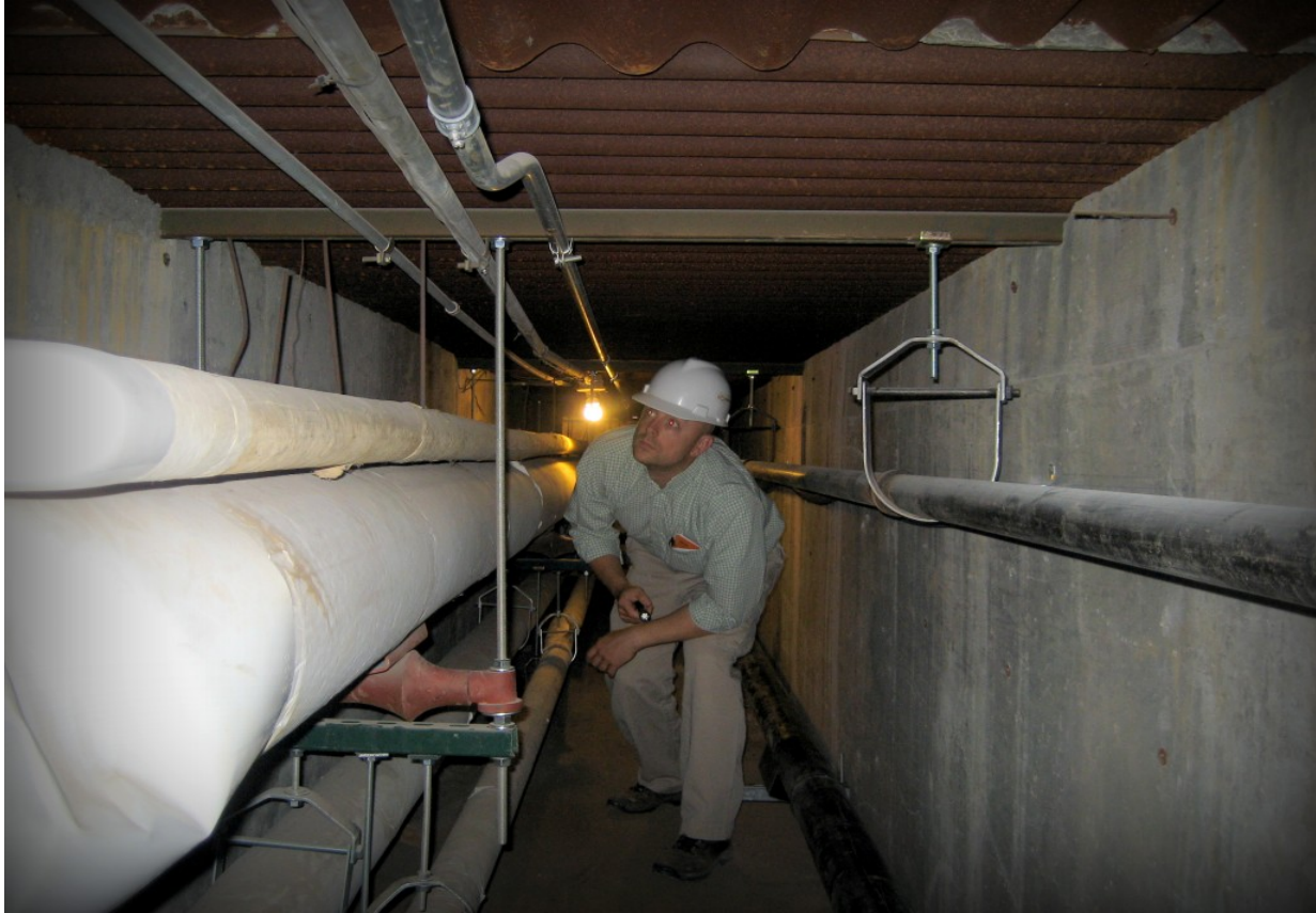
A commissioning agent inspects piping
