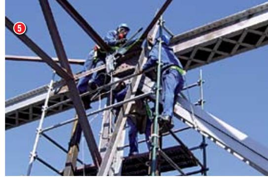
connections it was not possible to install a replacement member as a unit, and the four angle iron legs of the laced member had to be built up one by one.
