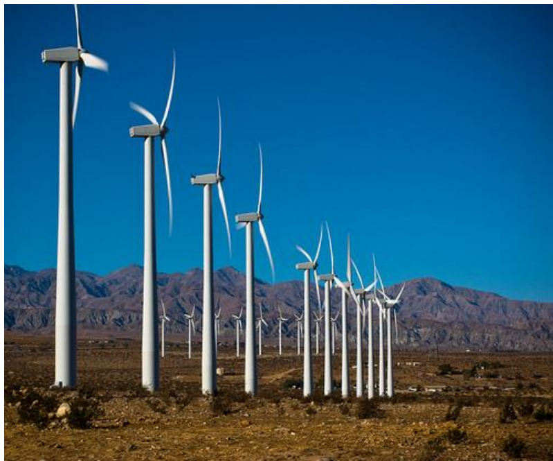
Wind Turbine Field (Palm Springs, CA)
