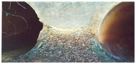
Concrete cancer in pipes Fernbank Creek, Hastings River floodplain, NSW 2001 The effects of acid sulfate soils on built environments may be more obvious. The ground may subside and lead to structural damage to roads, bridges and buildings.
