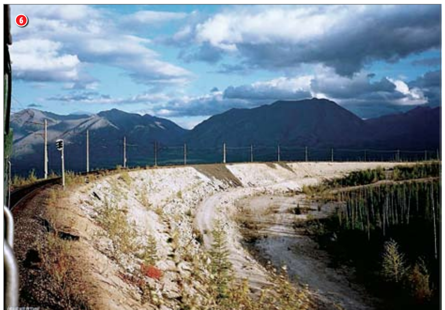
6 A section of the Severomuisk bypass
