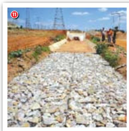
into streams adjacent to the development. The aim is to prevent flooding or damage to adjacent property, as well as to allow emergency vehicles to travel on internal roads.
