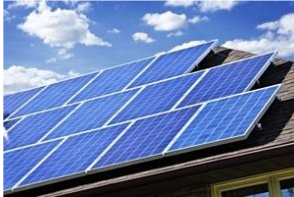
Residential rooftop installation of solar panels. US EPA
