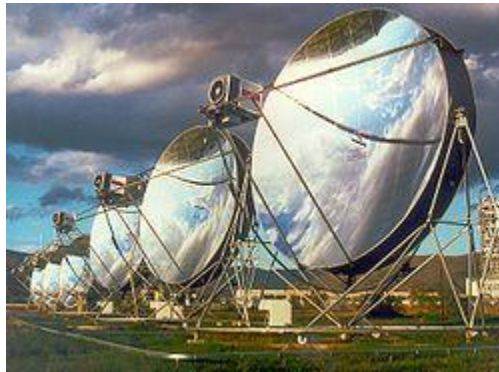
Stirling dish system at Plataforma Solar de Almeria, Spain. Source: Sandia National Laboratory
