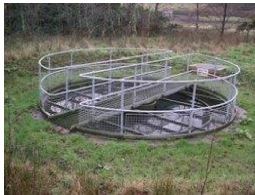
Secondary Sedimentation tank at a rural treatment plant
