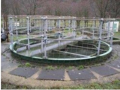
Primary sedimentation tank at a rural treatment plant
