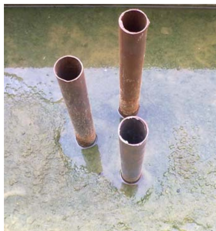
Figure 11. Scour hole around three piles with triangular arrangement
