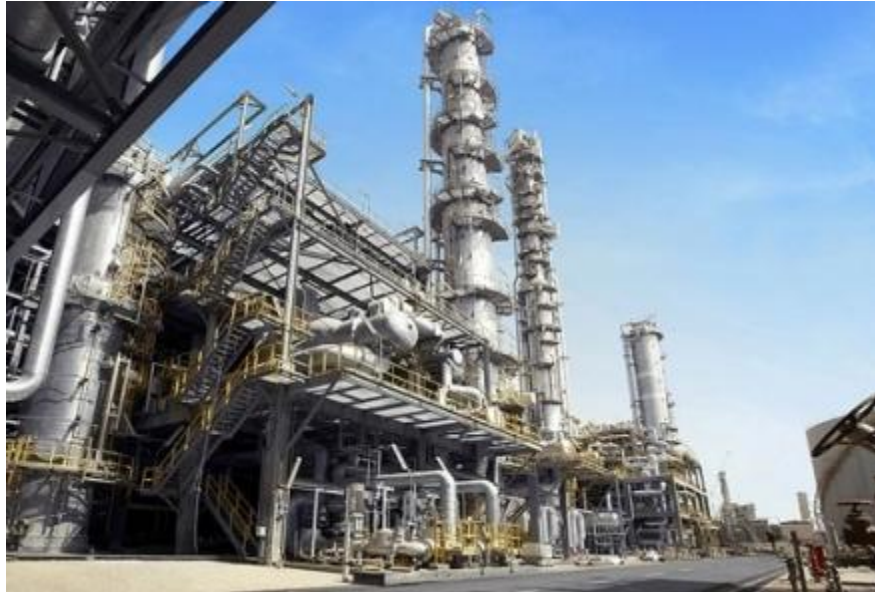
Saudi Arabian petrochemical plant. Source: Creative Commons
