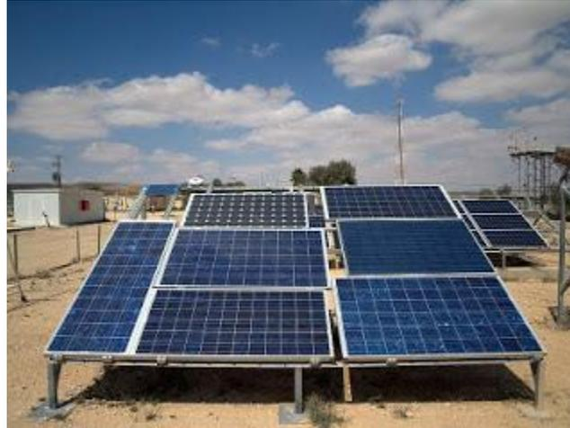
*A photovoltaic array is a linked assembly of PV modules.*
