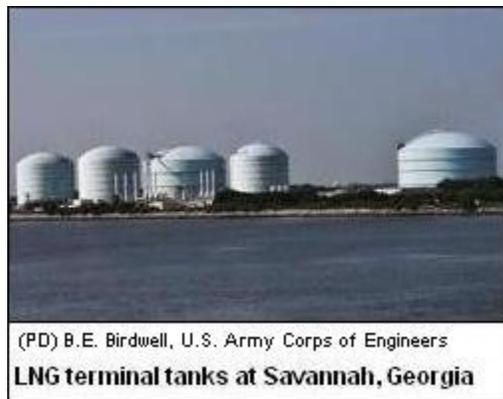
Large LNG storage tanks are cylindrical and have a low aspect ratio (i.e., height to width ratio). They are typically constructed with a post-tensioned concrete outer wall and a high-nickel steel inner wall, with insulation between the inner and outer walls. The tanks have domed roofs made of steel or concrete.
