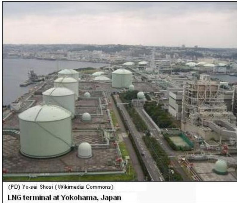
LNG receiving terminals (often referred to as "regasification terminals") receive LNG carriers, unload their LNG cargoes and store the LNG in tanks. When required, the LNG is withdrawn from the storage tanks, converted back into natural gas by using heat exchangers to vaporize the LNG, and then sent to the end consumers via a local pipeline grid.
