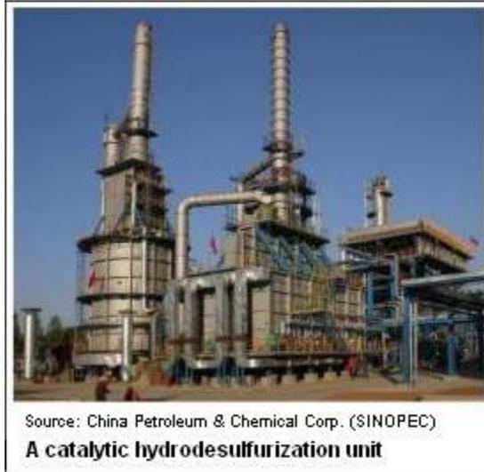
**Hydrodesulfurization** (HDS) or **Hydrotreating** is a catalytic chemical process widely used to remove sulfur compounds from refined petroleum products such as gasoline or petrol, jet fuel, diesel fuel, and fuel oils. One purpose for removing the sulfur is to reduce the sulfur dioxide emissions resulting from using those fuels in automotive vehicles, aircraft, railroad locomotives, ships, or oil burning power plants, residential and industrial furnaces, and other forms of fuel combustion.
