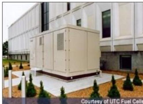
Stationary power is the most mature application for fuel cells. Stationary fuel cell units are used for backup power, power for remote locations, stand-alone power plants for towns and cities, distributed generation for buildings, and co-generation (in which excess thermalenergy from electricity generation is used for heat).
