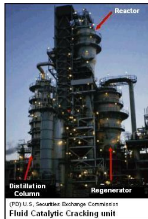
Suncor Denver petroleum refining facility features a fluid catalytic cracking unit.
