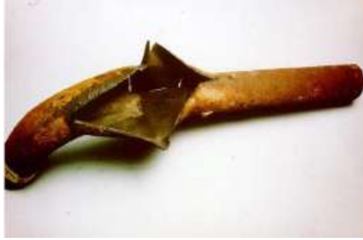
Figure 11: Ruptured CO 2 pipeline (Ø 130 × 8 mm) due to corrosion under insulation (CUI) (source: [9])
