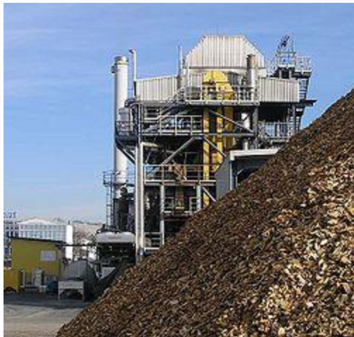
Wood chip gasification plant, Gussing, Austria
