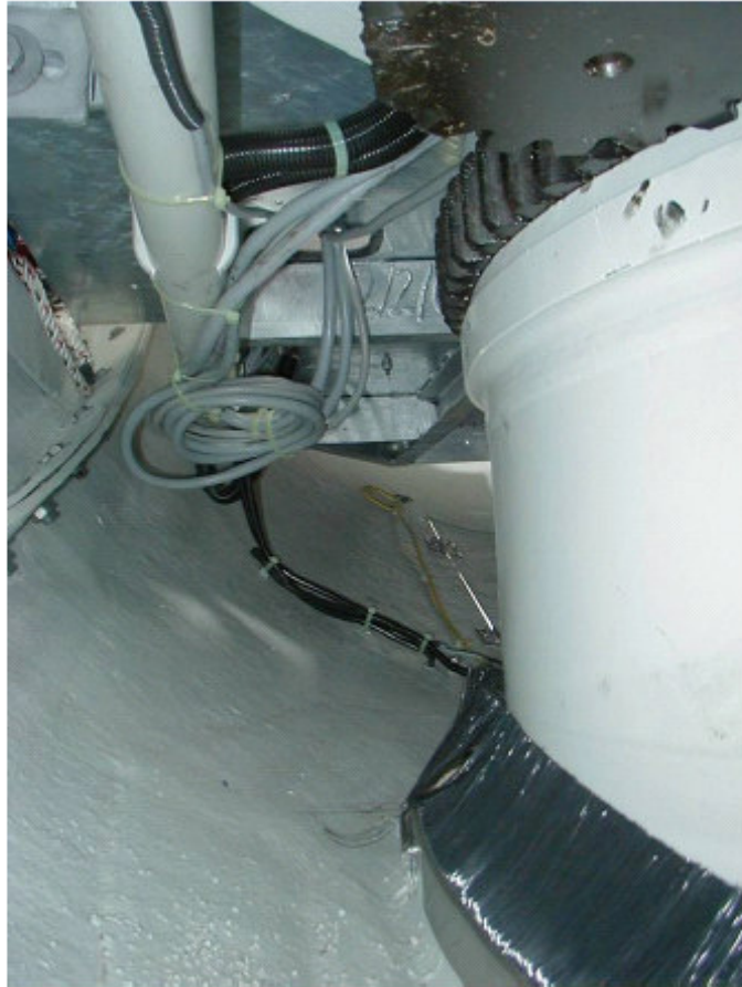
Figure 4 – Brush seals between the nacelle and tower
