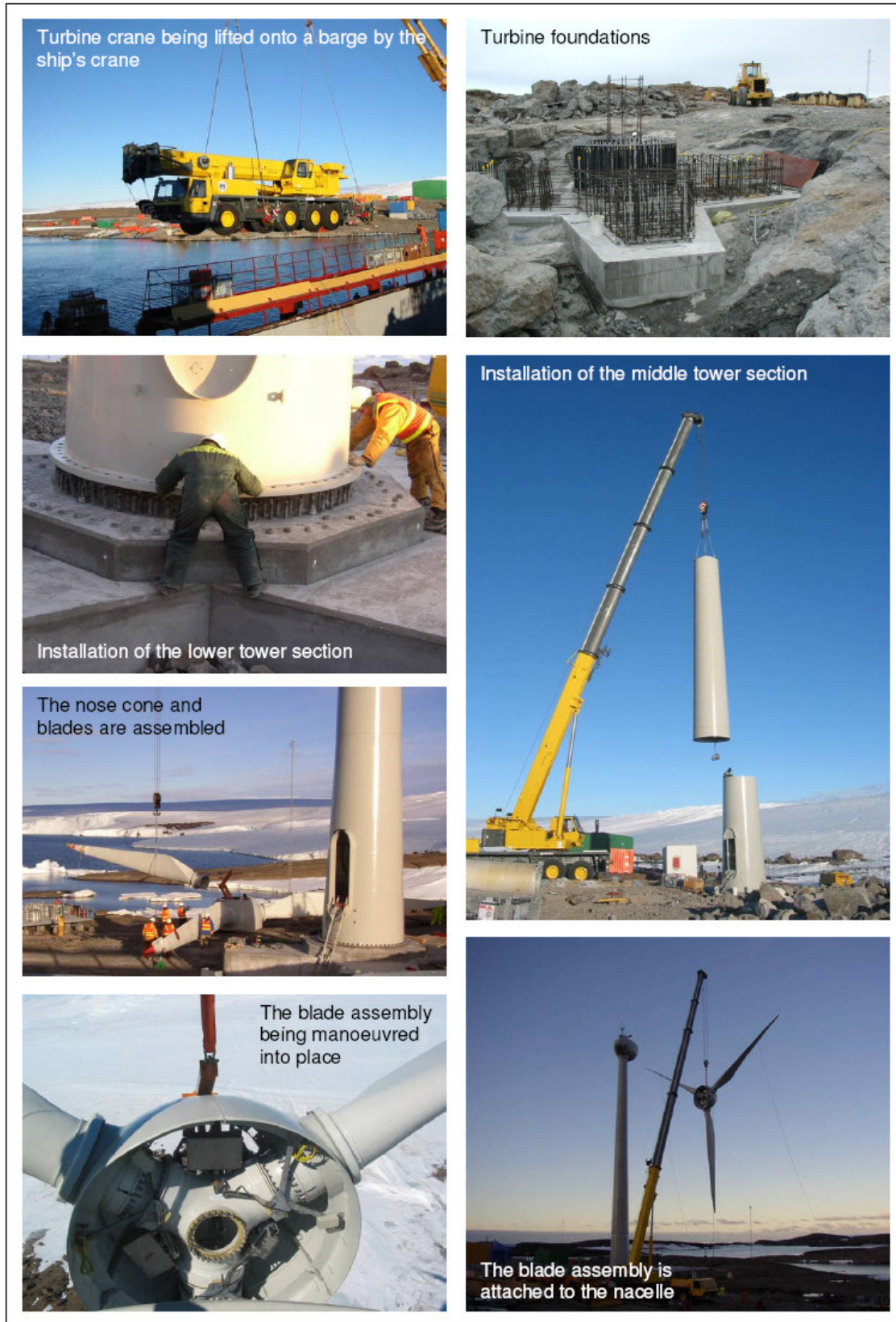
Figure 5 – Turbine installation
