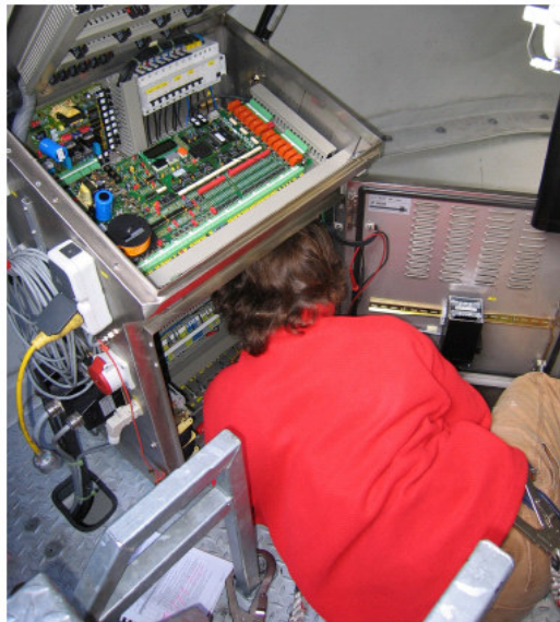
Figure 10 – At work in the nacelle
