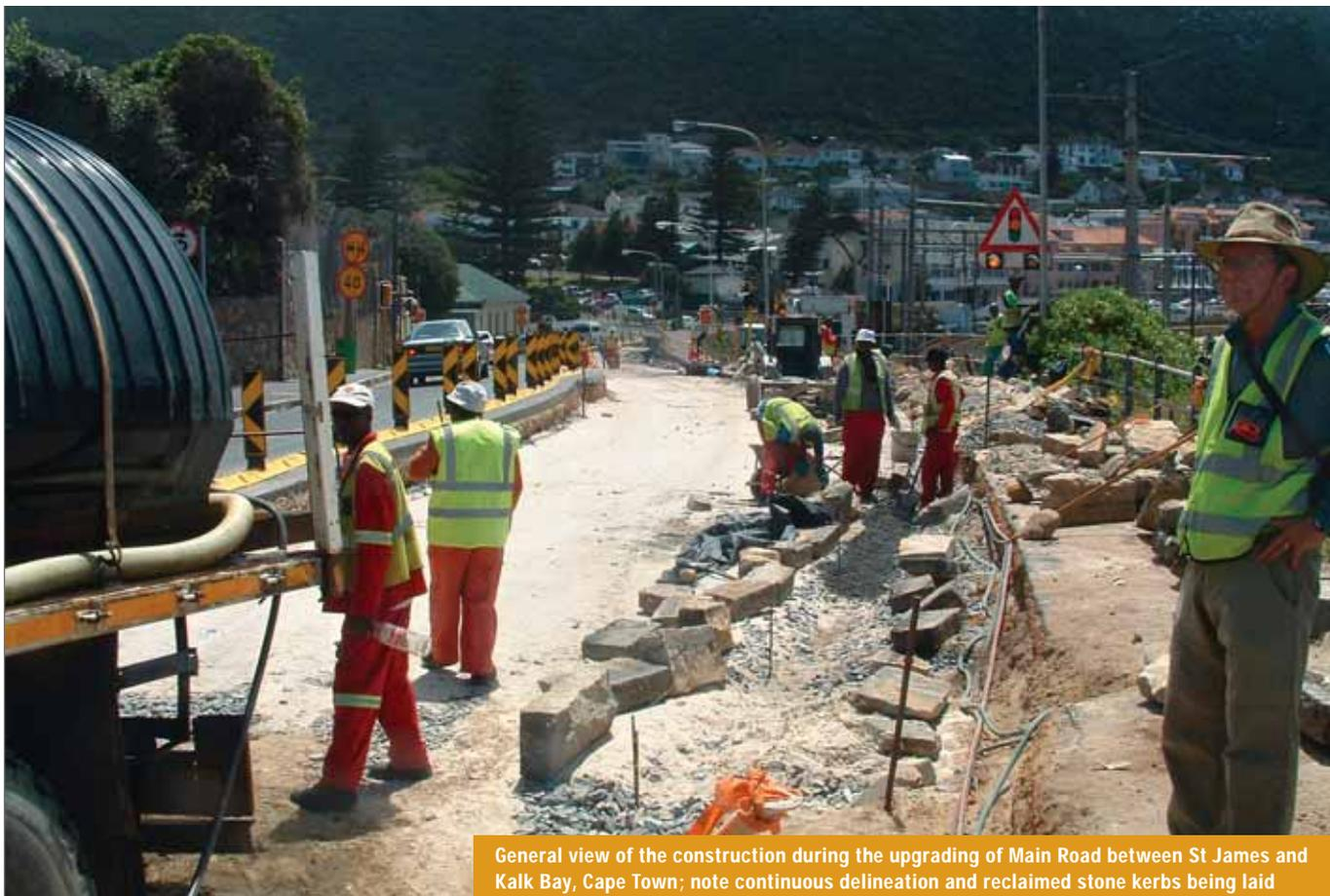
General view of the construction during the upgrading of Main Road between St James and Kalk Bay, Cape Town; note continuous delineation and reclaimed stone kerbs being laid
