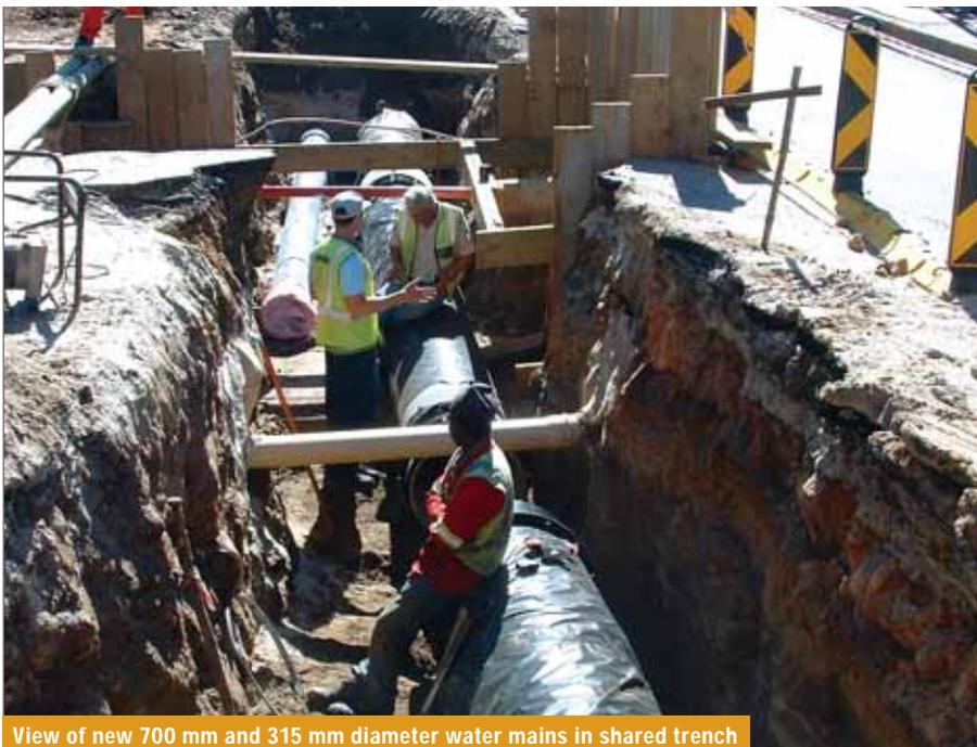
View of new 700 mm and 315 mm diameter water mains in shared trench
