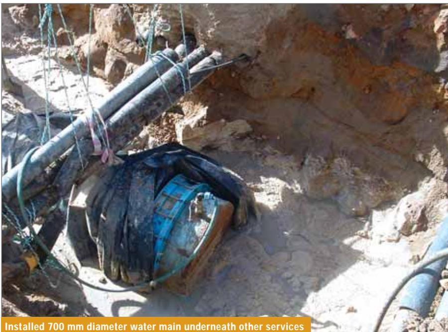
Installed 700 mm diameter water main underneath other services
