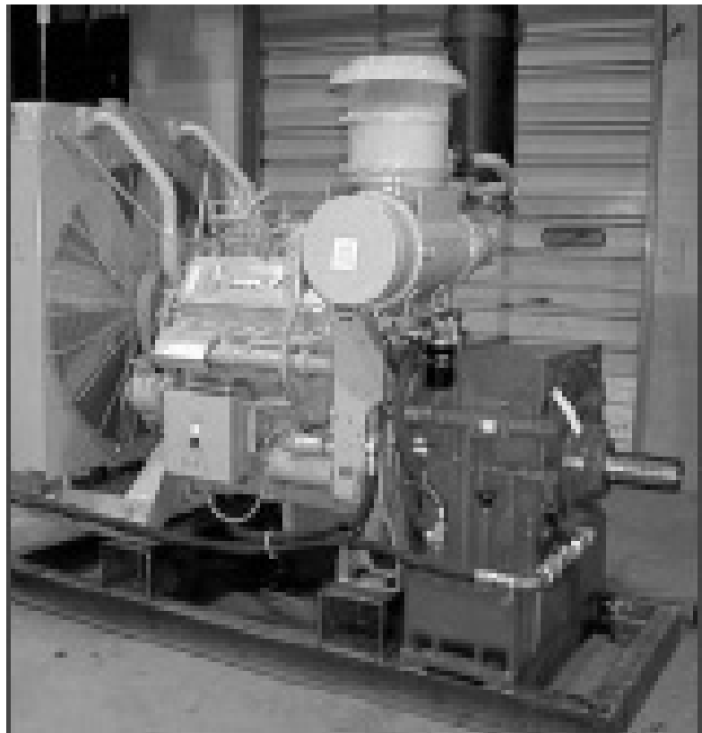
Fig 1.5 An Industrial skid mounted Diesel Generator
